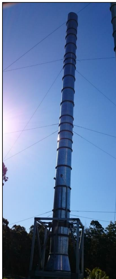
Figure 4-1: EPL Point 3 (Wet Separator Stack)
