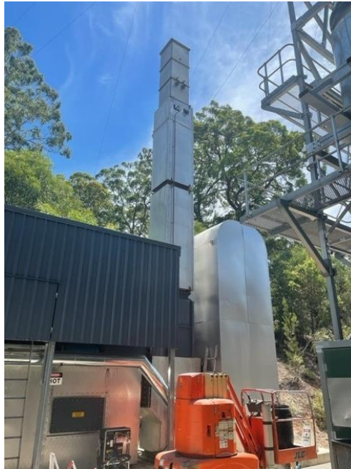
Figure 4-3: Regenerative Thermal Oxidiser Stack
